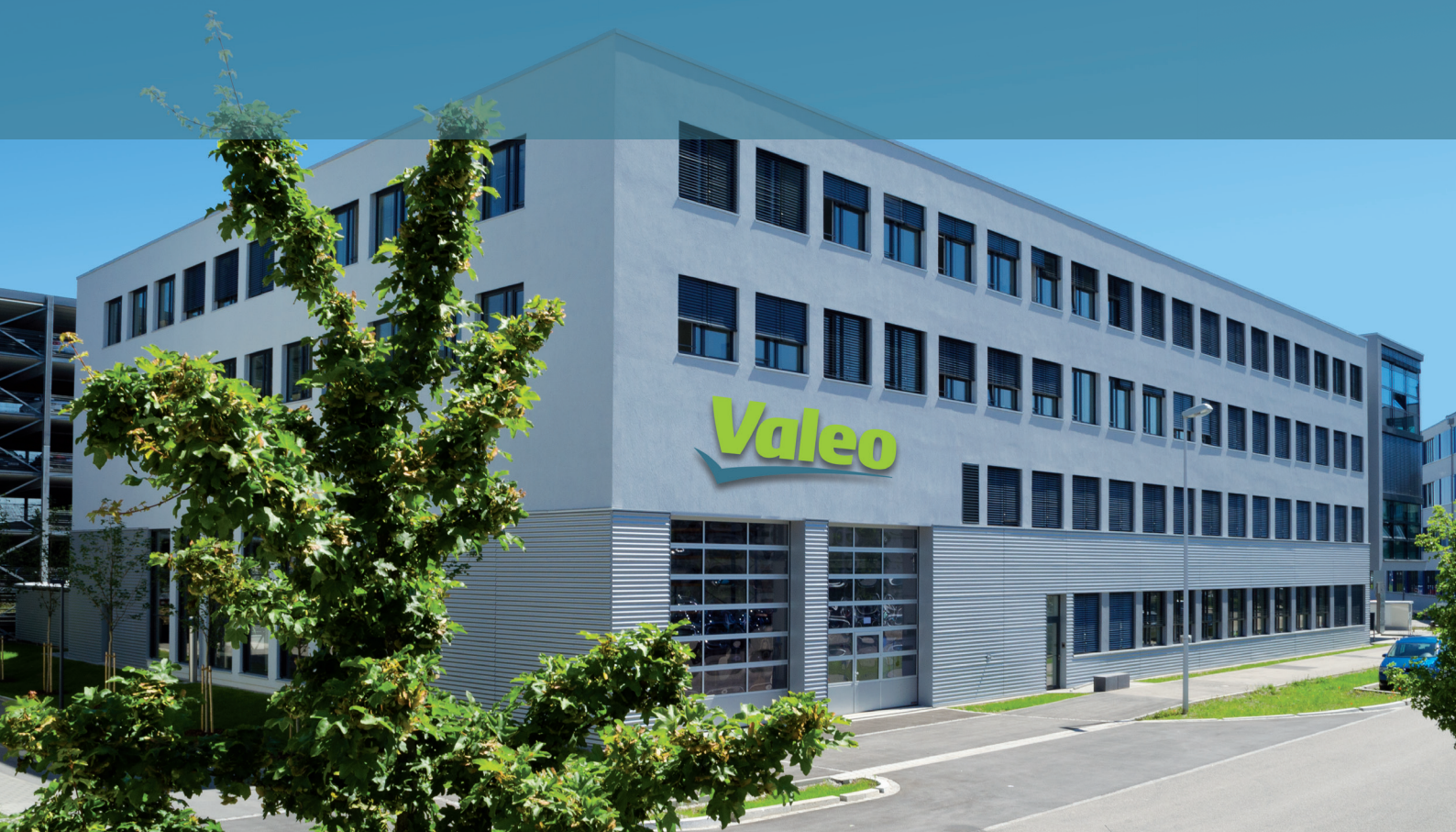
Technology centre at the Gilching facility in Germany.
